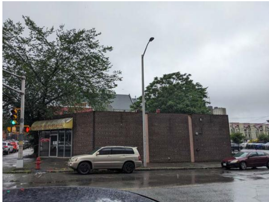
Existing Building on Block 2
